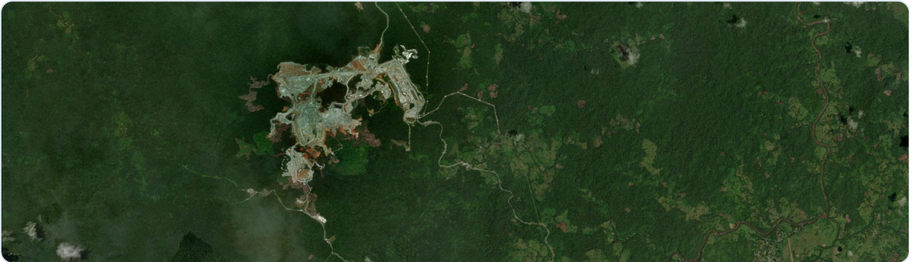
COBRE PANAMÁ, DONOSO DISTRICT, PANAMA. THE OPEN PITS, PROCESSING PLANT AND TAILINGS FACILITY UNDER PRESERVATION & SAFE MANAGEMENT. IMAGERY: ESRI WORLD IMAGERY (MAXAR / EARTHSTAR).
